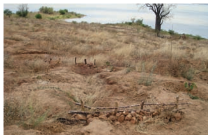
Anti-erosion measures: Checkdams constructed with sticks and stones, along the course of a gully, and a gully showing the extent of soil being washed away.
